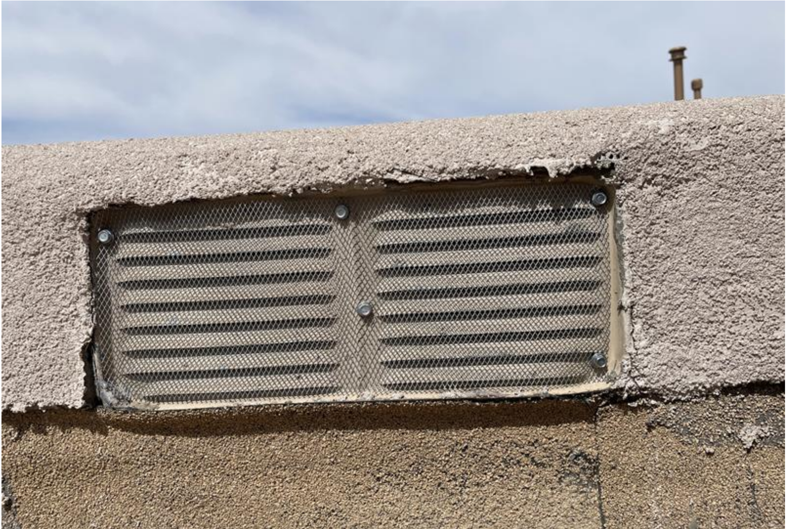
KwikMesh 1/8" stainless steel wire screen over existing louvered parapet vent
